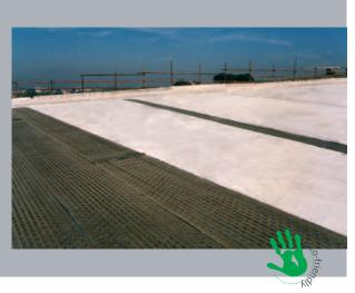
**PROJECT SPECIFICATIONS**: regulation element used on roofing where the membrane is partially bonded and when a vapour barrier and thermal insulation is installed.
